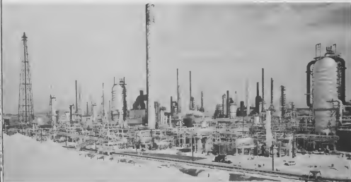
Lago's HDS Facilities.
